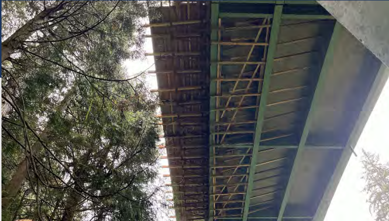
Falsework installed
