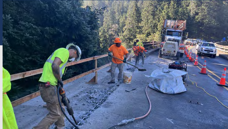
Chipping guns used to remove concrete
